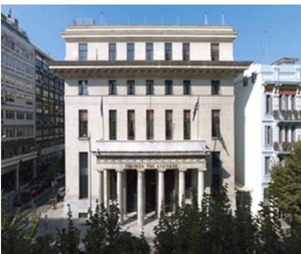
Bank of Greece building- Thessaloniki
